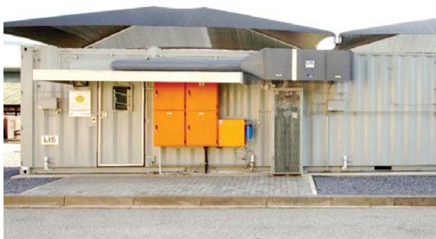
The newly built plant containment facility. The building management control system and switches are housed within the distribution boxes (larger orange units) and linked with WiFi to the main Biotechnology Platform building from which this photo was taken. Climate control features, such as the carbon dioxide supplementing tanks and relays, humidification system and its relays (smaller orange unit), as well as the air treatment unit (large ducting) are visible in this front view. All the air conditioning and other utilities are cleverly hidden under corrugated cover plates. Heat reflective paint on the roof and 80% shade cloth helps with passive energy conservation.
