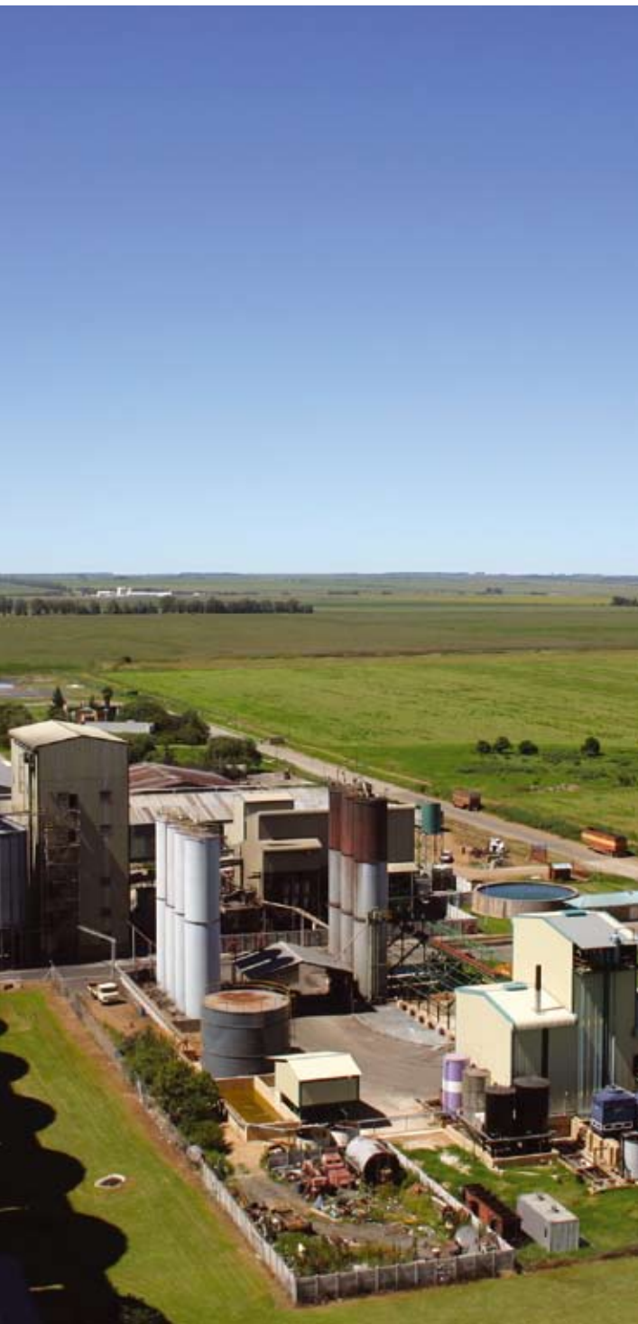
NWK's Lottiehalte silo and Epco sunflower seed crushing and extraction plant. Photo: NWK
