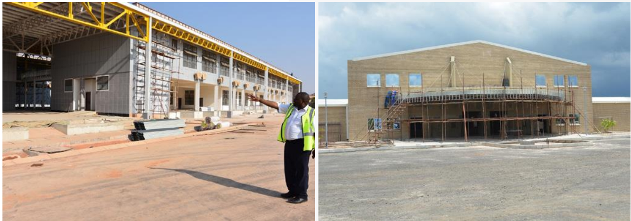
Figure 11 – OSBPs under construction at Mwami and Kazungula, Zambia
