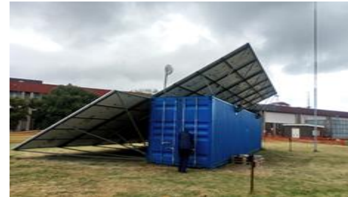
Containerised microgrid
