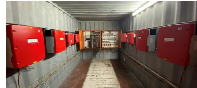
Containerised microgrid
